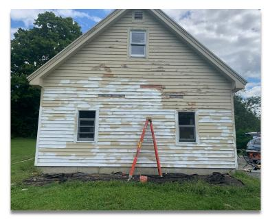
The peeling paint wasn't just an aesthetic issue; it posed serious risks. Homes with deteriorating paint are more susceptible to moisture infiltration, which can lead to mold growth, wood rot, and structural damage over time. Similarly, the hole in Ruth's siding could have caused havoc: squirrels nesting inside homes can chew through wiring, cause insulation damage, and even create fire hazards.
